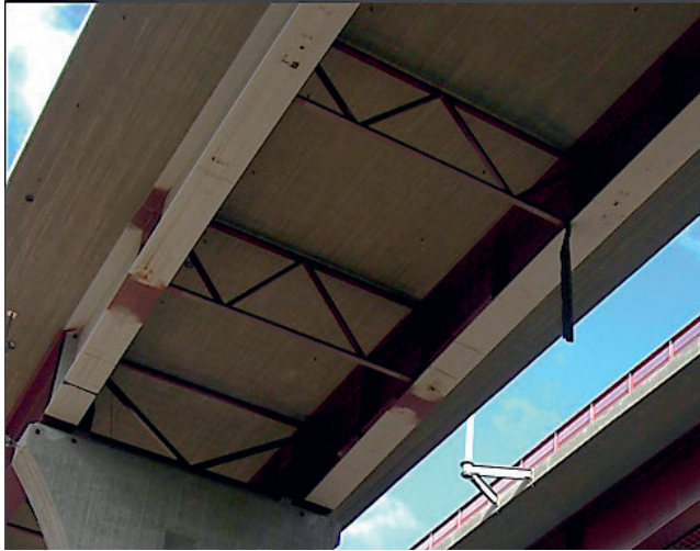
Figure 20 Pair of vertical K-bracing. Source: Heikki Lälja
