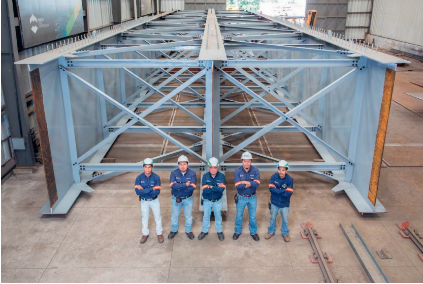
Figure 27 The Oxec Bridge in Guatemala. Source: PEDELTA
