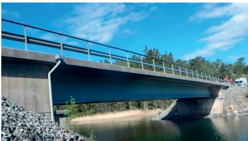
Figure 31 The Yxlö Bridge in summertime. Source: The Swedish Transport Administration, n.d.
