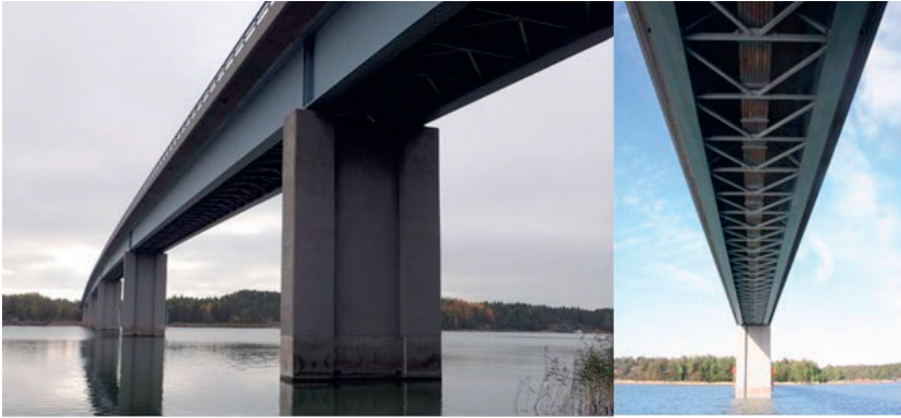
Figure 22. Kaitainen bridge. Source: Heikki Lilja
