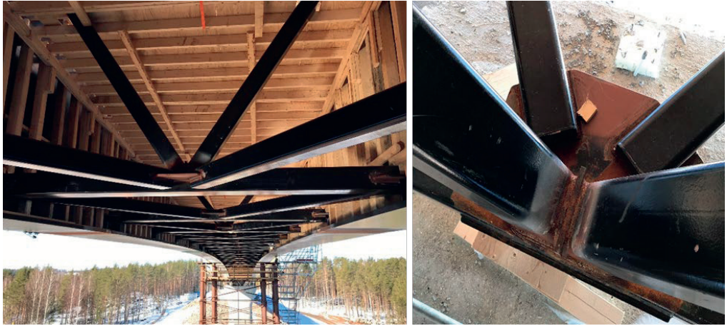
Figure 9. Connections between the horizontal and vertical bracing at Vekaransalmi Bridge.
