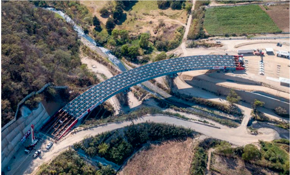
Figure 14. Launching nearly completed.
