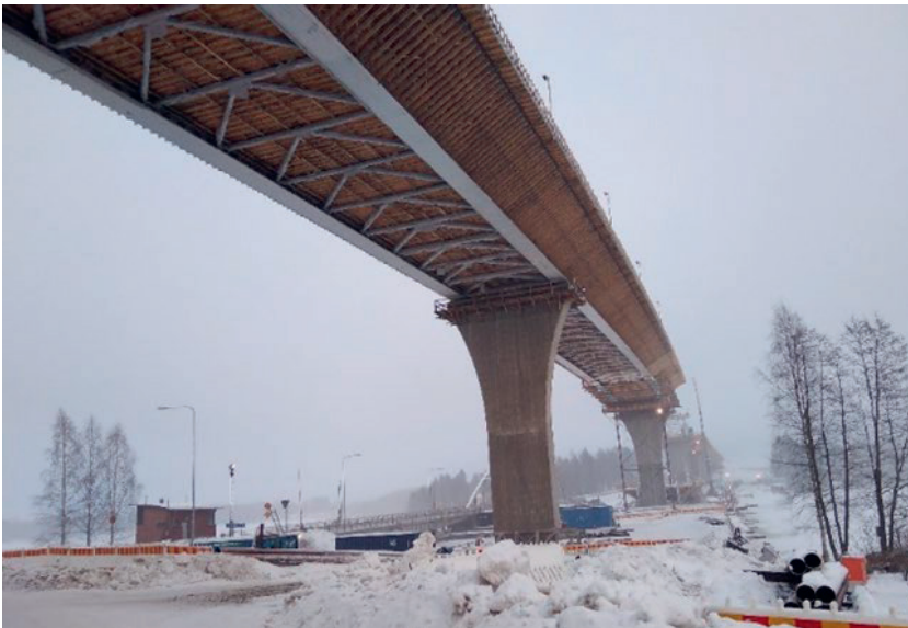
Figure 23. Jännevirta bridge. Source: Ramboll
