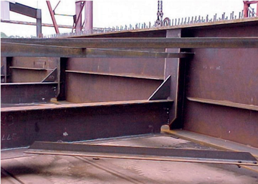
Figure 25. Bottom lateral bracing between the bottom flanges and temporary bracing at the top part of the girders. Source: Jacques Berthelémy
