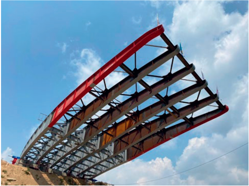
Figure 13. Initial launching of bridge 15 over Pinulla River
