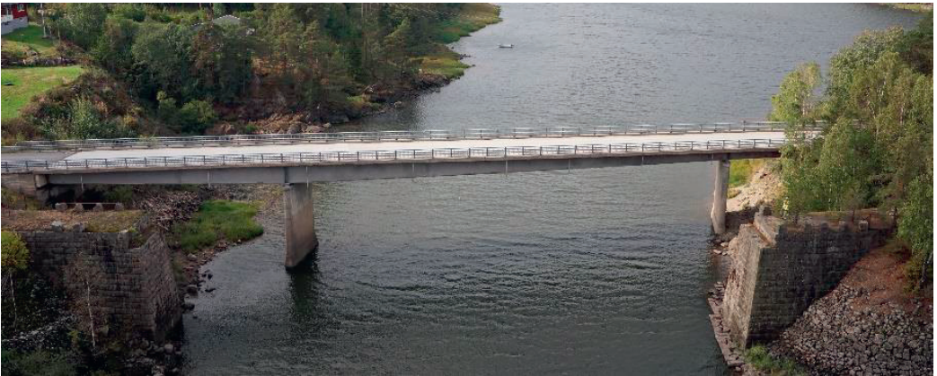
Figure 1. Overview of bridge location, taken from north
