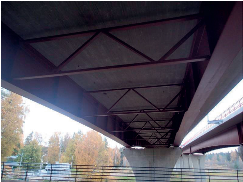
Figure 8. Cross bracings in the Mälkiä channel bridge A
