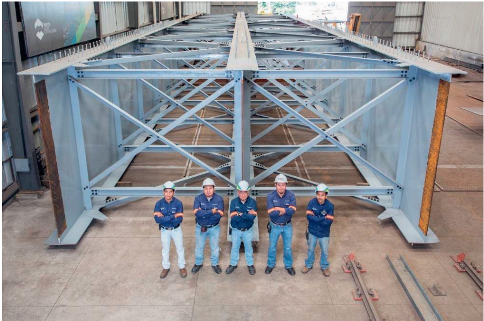
Figure 12. Oxec Bridge in the workshop.
